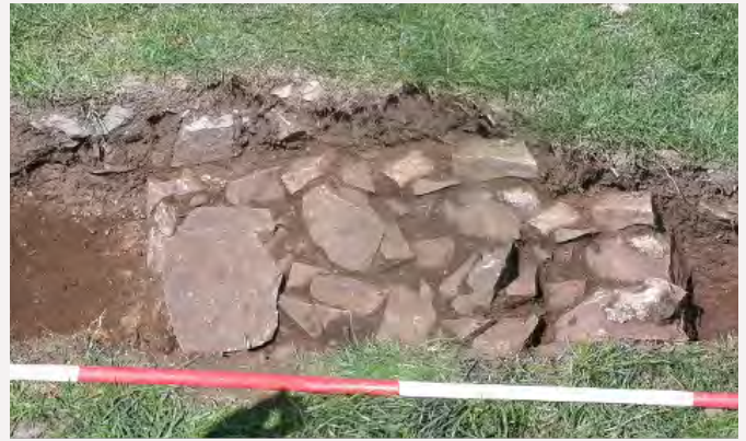
Trench 2 showing mortared wall underlying stone 'garden bank'
