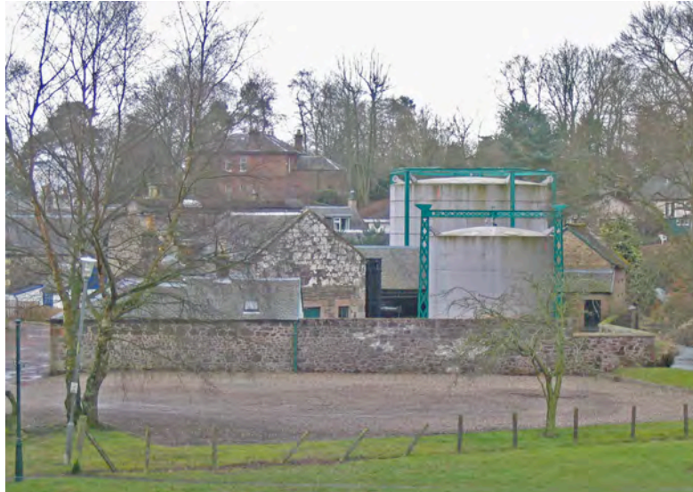
Pl 21. Biggar town gasworks, the only example left in Scotland - open to the public.
