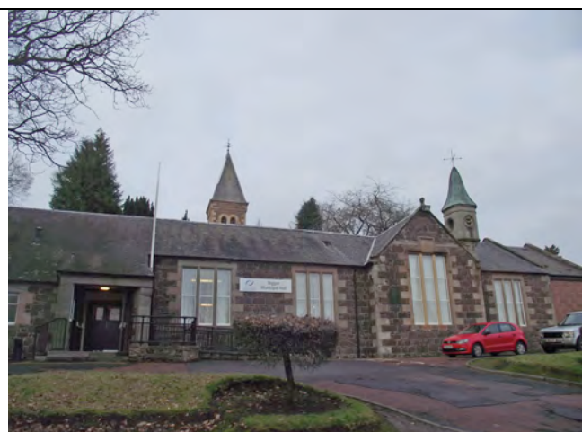
PI 36. The new Parish School and later town hall. With later additions at each end.
