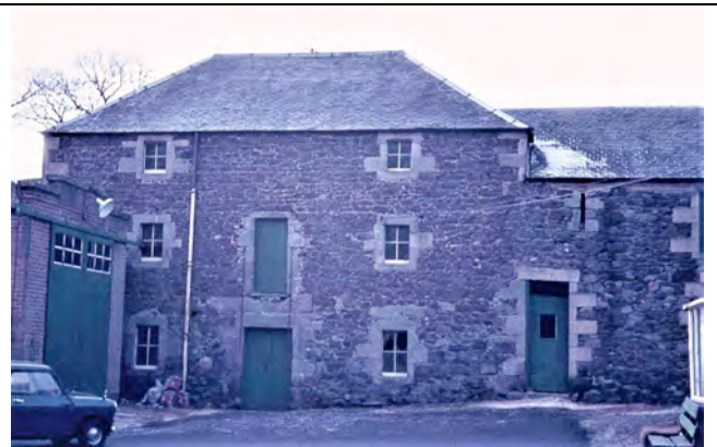
Pl 23. Biggar Corn Mill, currently being converted to housing.
