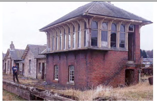
Pl 17. Biggar Station signal box.
