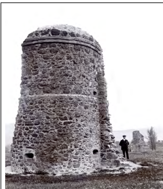
Pl 13. Boghall tower after preservation 1912. Note the gun ports.
