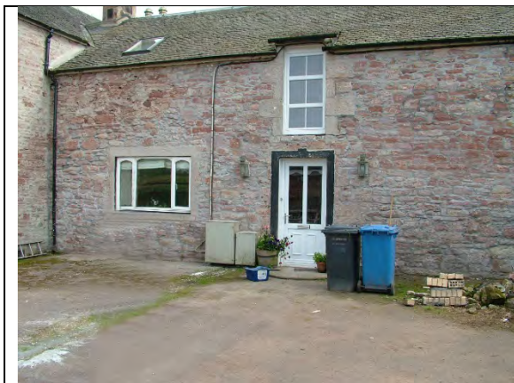
Plate 1. Showing east end of north wall with former upper floor doorway
