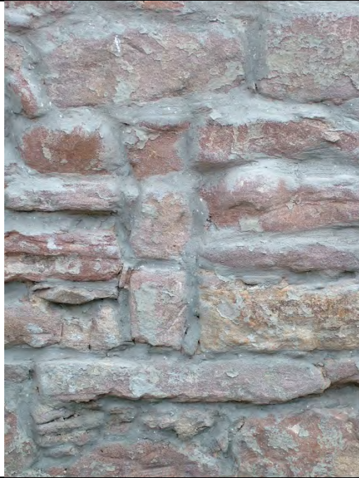
Plate 4. Showing blocked slit window
