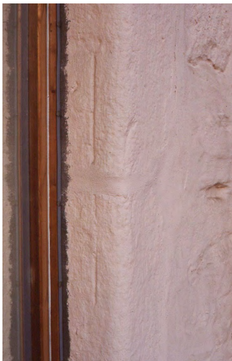
Plate 8. Showing window stones with glazing slots, now re-used in a doorway.
