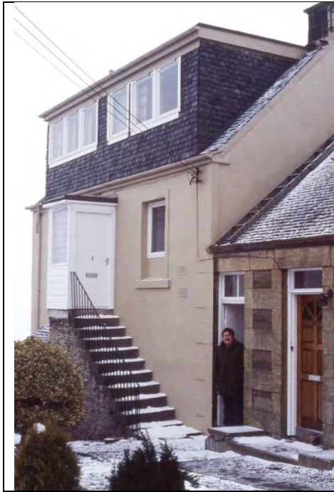
Plate 9. Showing building on first day visit
