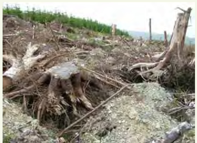
Borrow pit back filled with tree stumps
